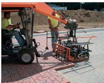
The Eco-Stone® Family of Permeable Pavers features shapes that offer the highest degree of interlock and have been tested and proven worldwide. They are designed for fast mechanical installation, saving time and money on construction, and when
