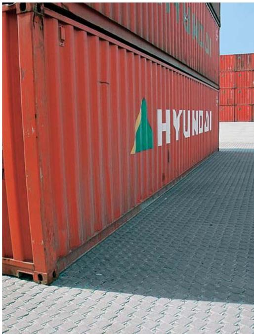
UNI<sup>®</sup> Permeable Pavers are very effective at reducing the volume of stormwater runoff and its associated pollutants through infiltration and detention. They are ideal for areas where storm sewers are at capacity, where detention or retention ponds are not feasible, when groundwater recharge is a priority due to population demands or drought, and in areas where impervious cover is restricted.
